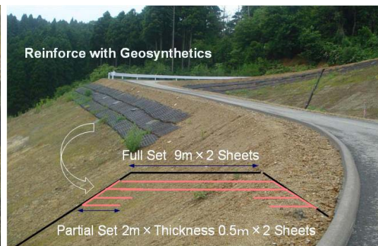
Crest Reinforcement at Road Bank
