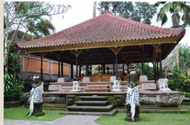
`Pendopo` as part of architecture traditional Bali
